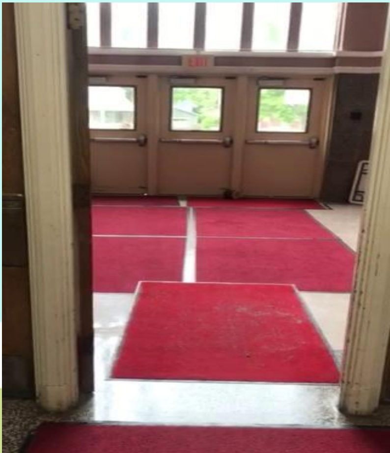
Main Hallway & Office
